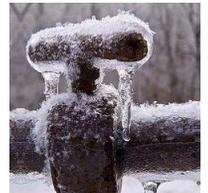
Also be sure to insulate the metal fittings, such as the relief valve, ball valve, hose bibb, check valve, and pressure gauge. For the items you want to be able to get to later (such as the pressure gauge and hose bibb) make a glove out of the pipe insulation that will tightly slip down over the item when not in use.
